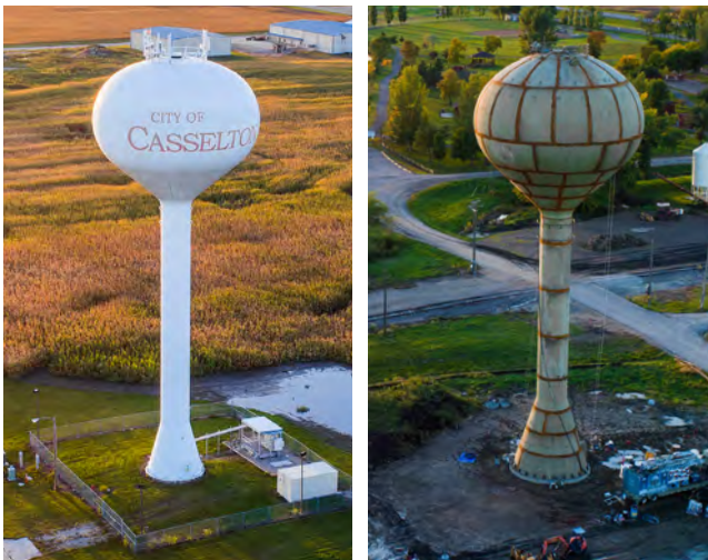
Fig. 6.7 | Existing Water Tower New Water Tower
