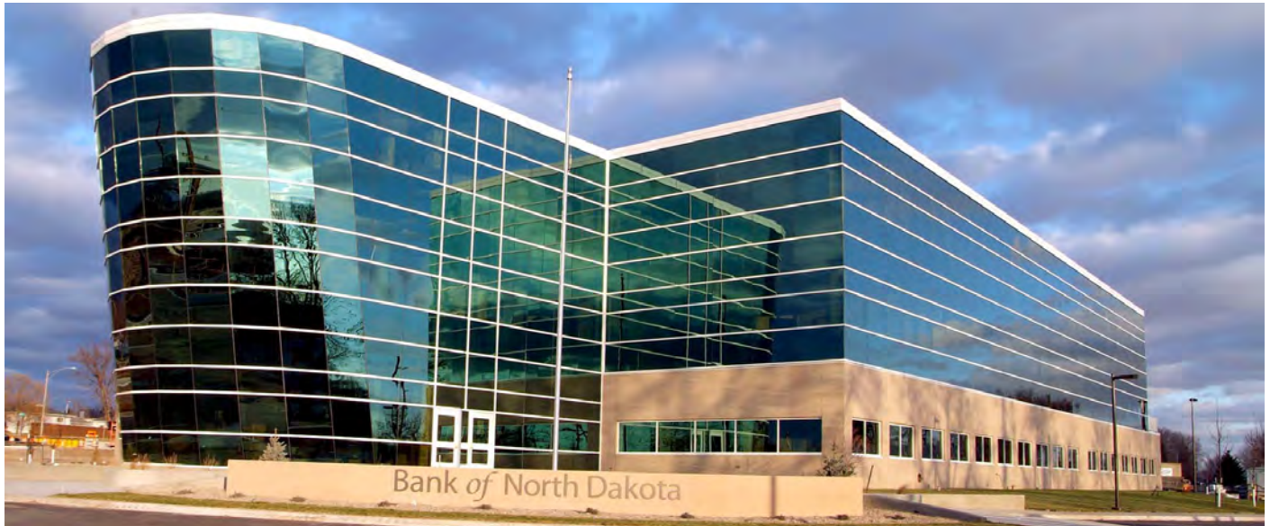
Fig. 8.1 | Bank of North Dakota Headquarters, Bismarck
