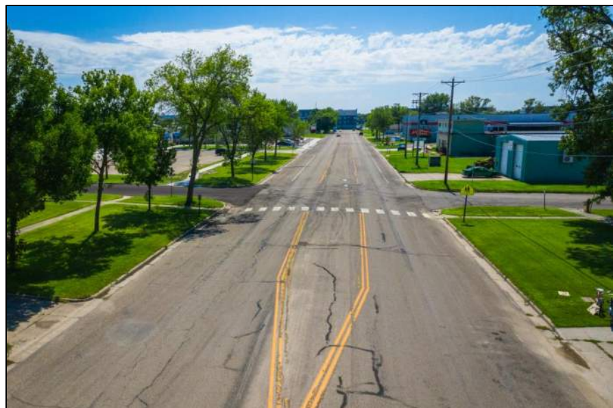
Transition from three-lane to two-lane section near 4th Ave N
