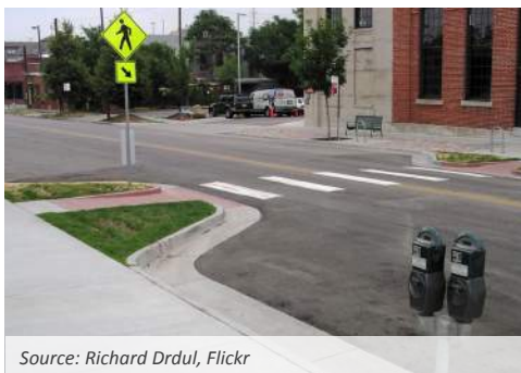
ABOVE Permanent bumpout: full reconstruction
