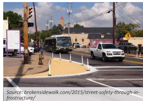
ABOVE Temporary bumpout: mill and overlay
