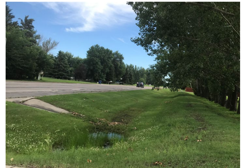
Ditches and stormwater infrastructure along the west side of 11th Street North.
