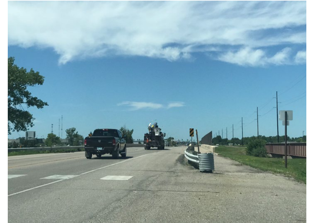
Existing conditions on US Highway 52 near 34th Street, looking north.
