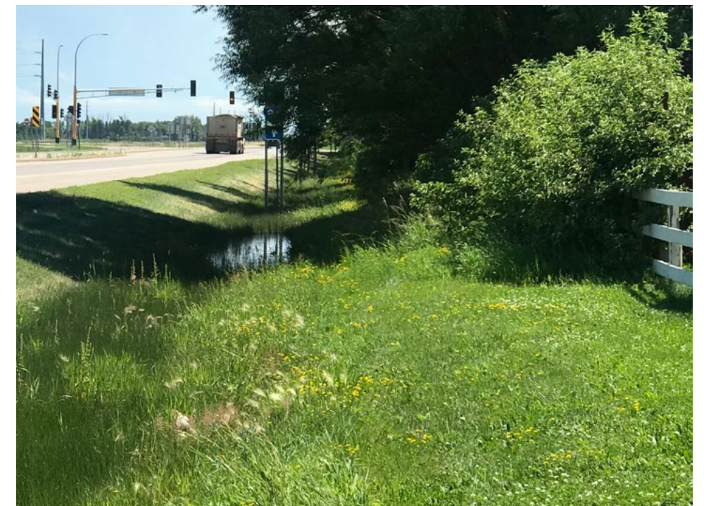
Deep ditches on the side of US Highway 52 near 29th Avenue South.
