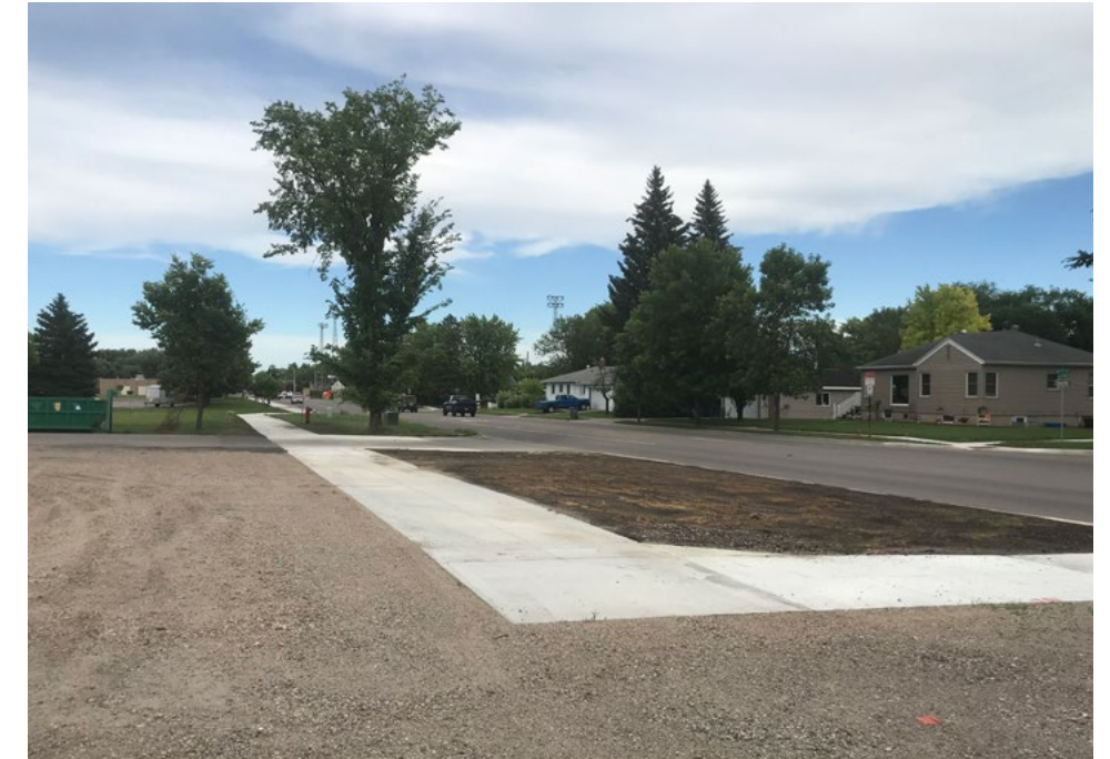
A shared use path that was recently constructed along the north side of 15th Avenue North, which connects to the southern terminus of Gap 16.
