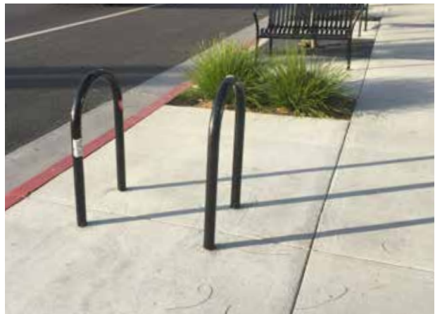
Inverted-U racks provide two points of contact.
