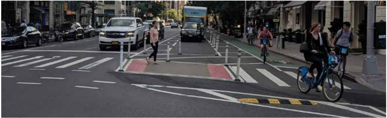
Parked cars serve as a barrier between bicyclists and the vehicle lane. Barriers could also include flexible posts, bollards, planters, or other design elements. Source: Alta
