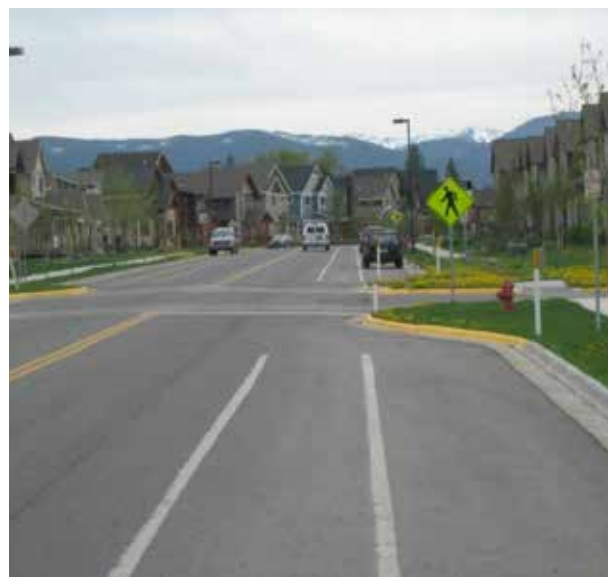
Vertical delineators help inform snow plow drivers of obstacles such as cycletracks, raised medians and bulb-outs in Salt Lake City, UT
