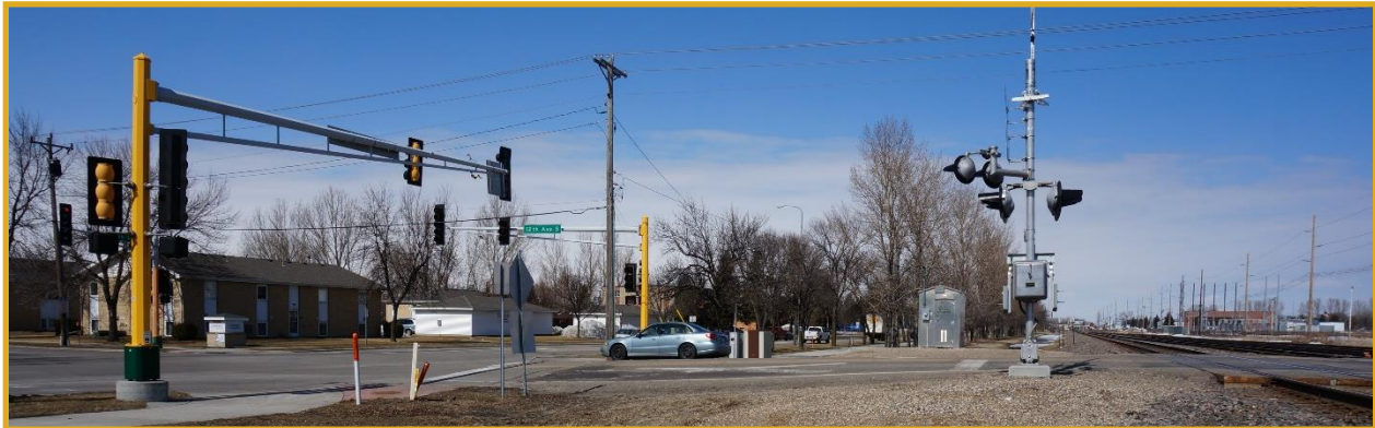
20th Street South Intersection, Facing North
