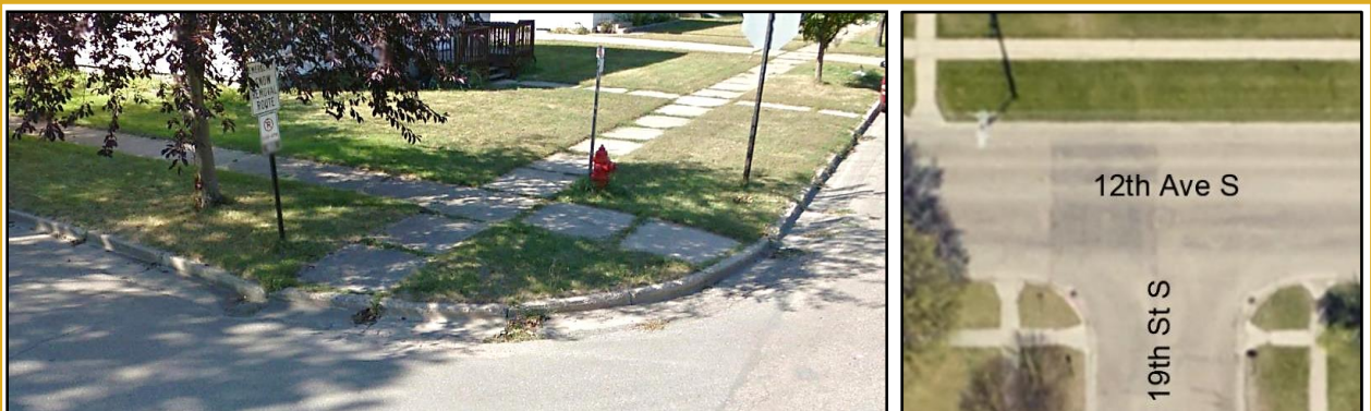
Many Sidewalk Curb Ramps Do Not Meet Current ADA Guidelines or Do Not Align
