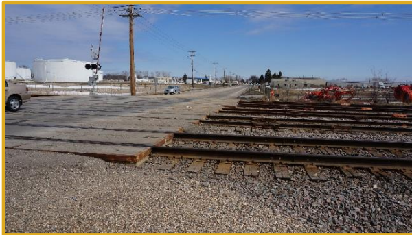
BNSF RR Crossing east of 20 th Street
