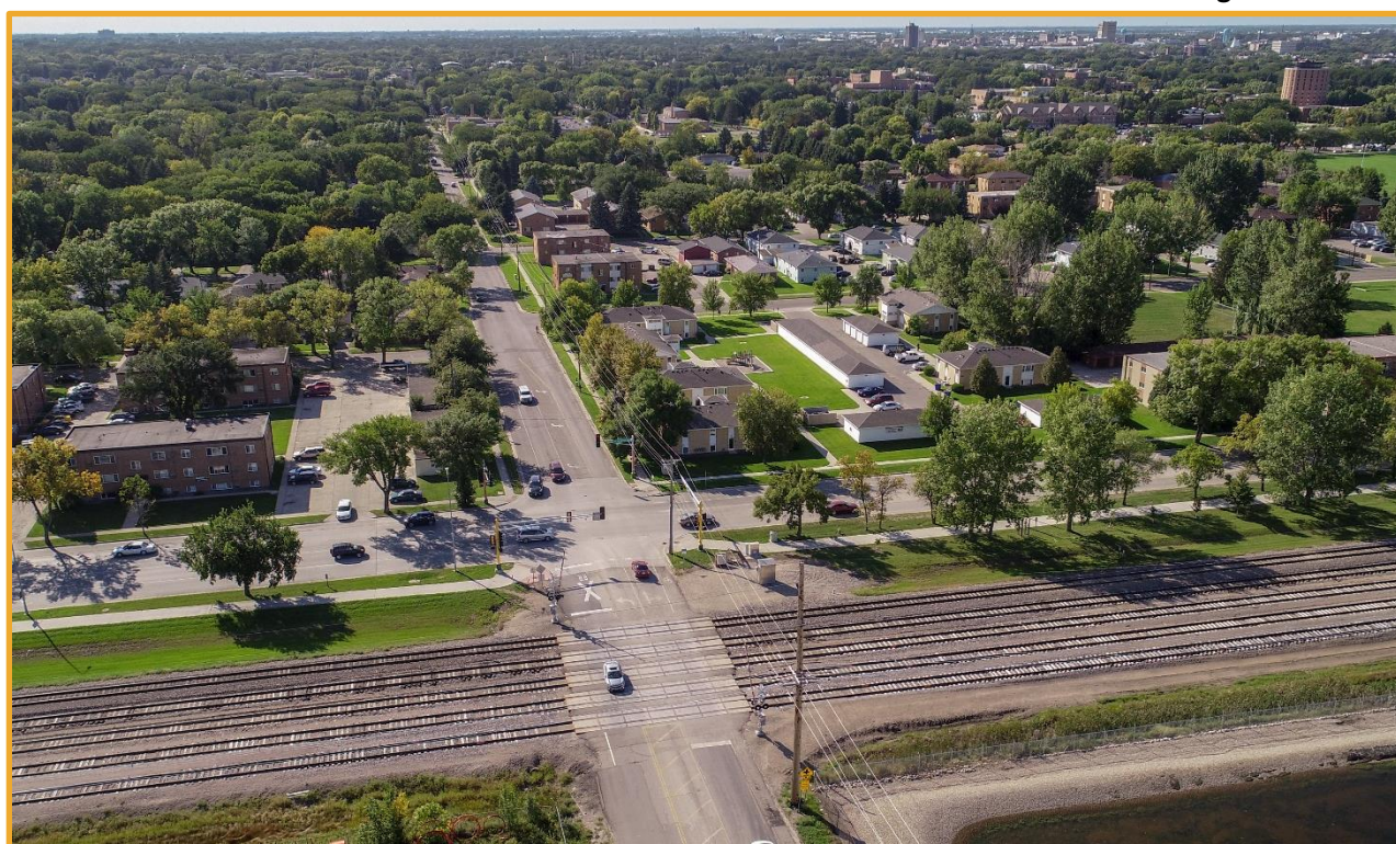
Railroad Crossing at 20 th Street
