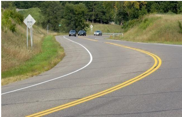
Figure 3-6. Shoulder Paving
