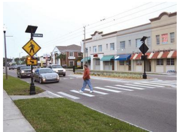
Figure 3-14. Rectangular Rapid Flash Beacon (RRFB)
