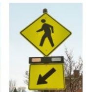
Rectangular Rapid Flashing Beacon
