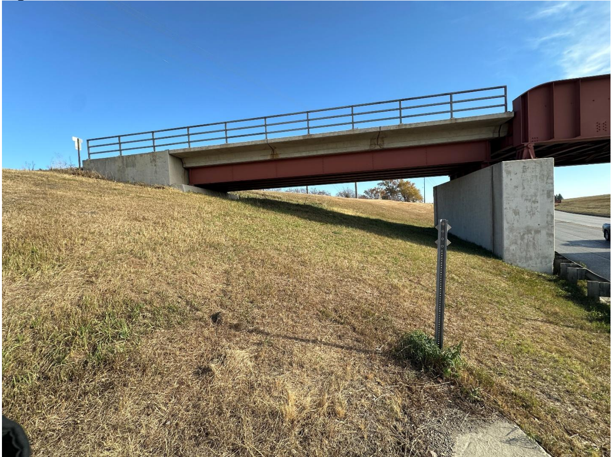
Northwest side of crossing looking East
