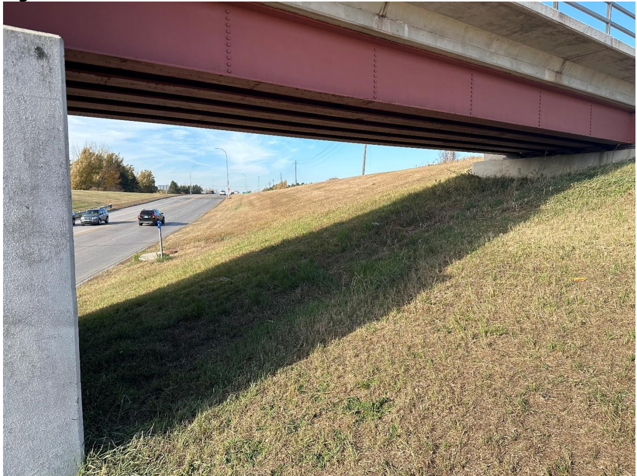
Northeast side of crossing looking West
