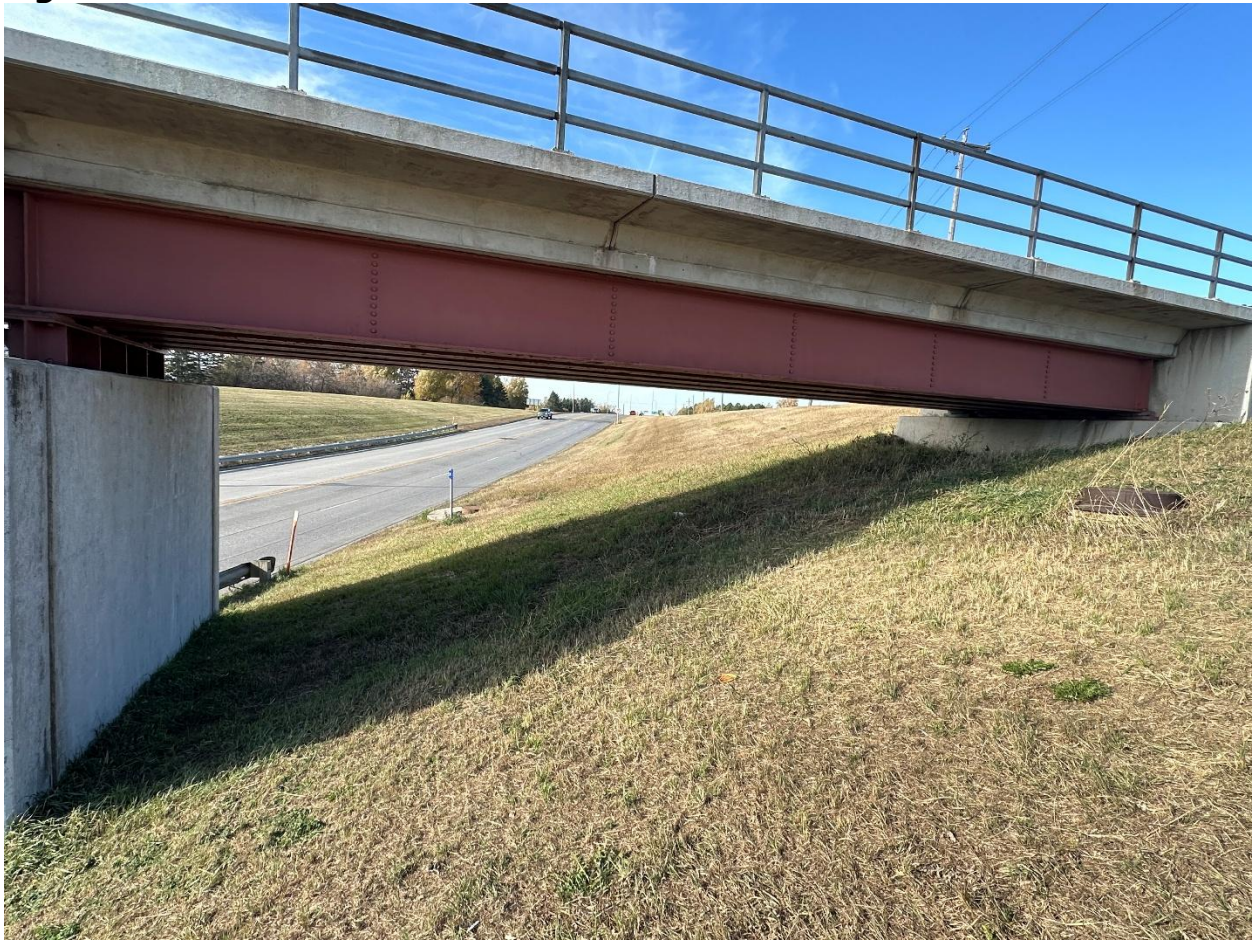
Northeast side of crossing looking West
