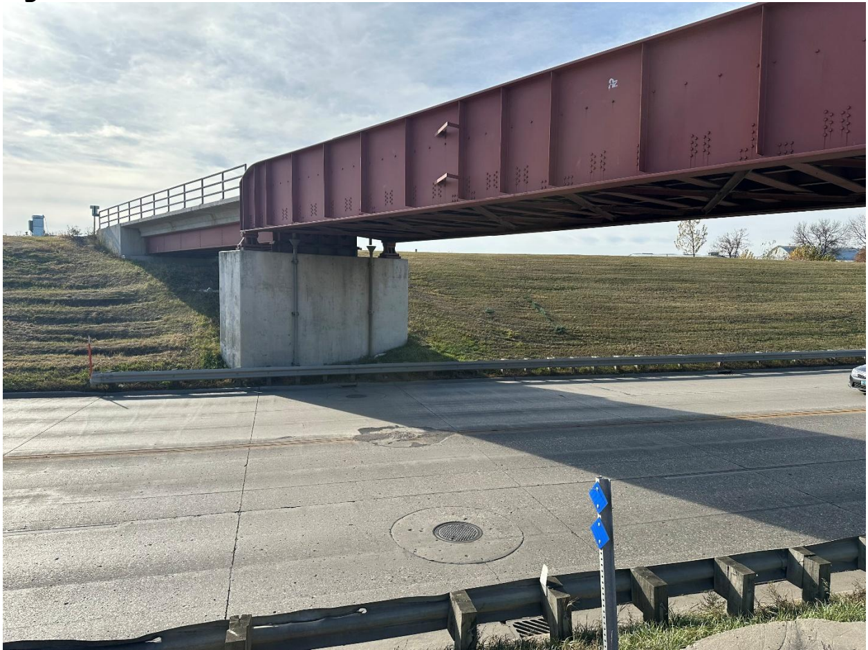
Northeast side of crossing looking South
