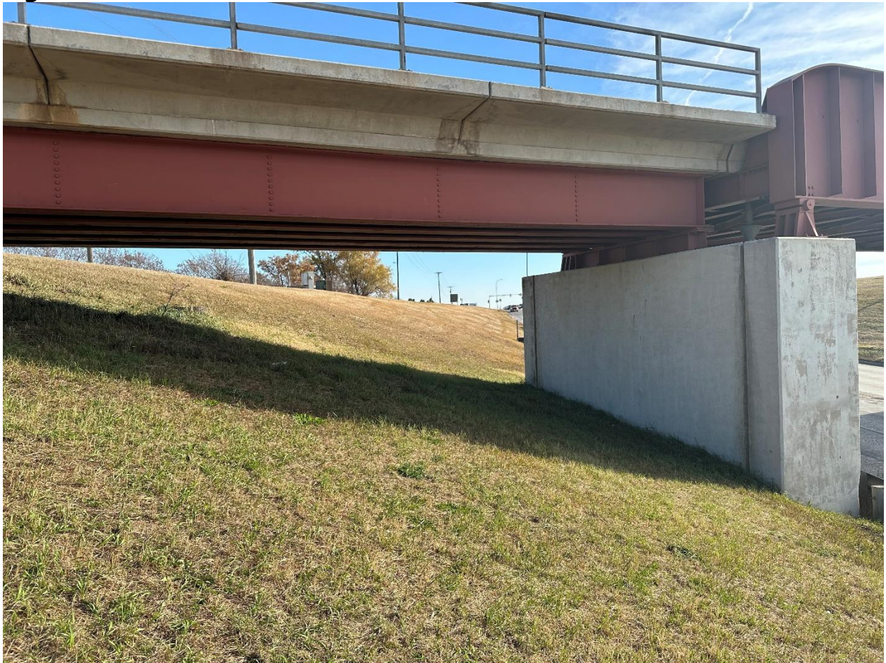
Northwest side of crossing looking East
