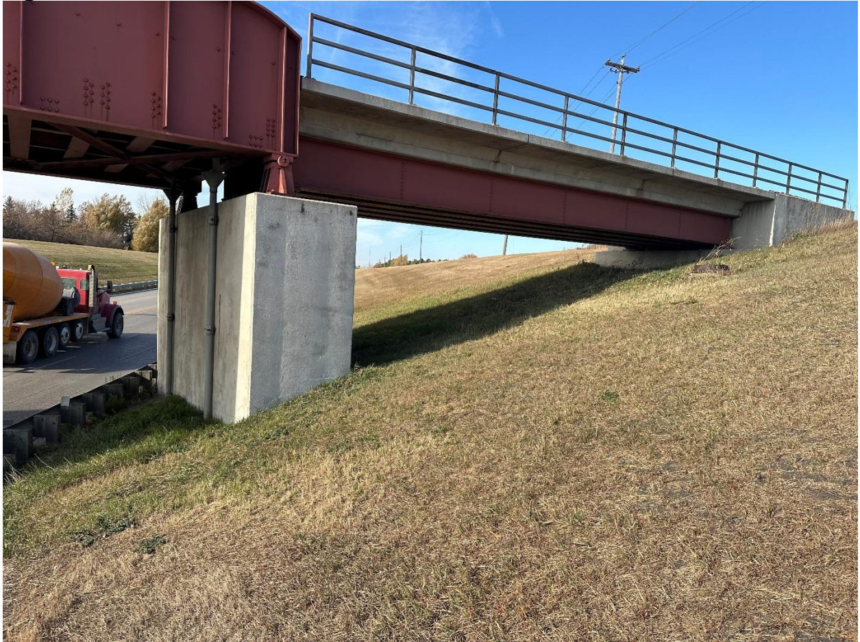
Northeast side of crossing looking West
