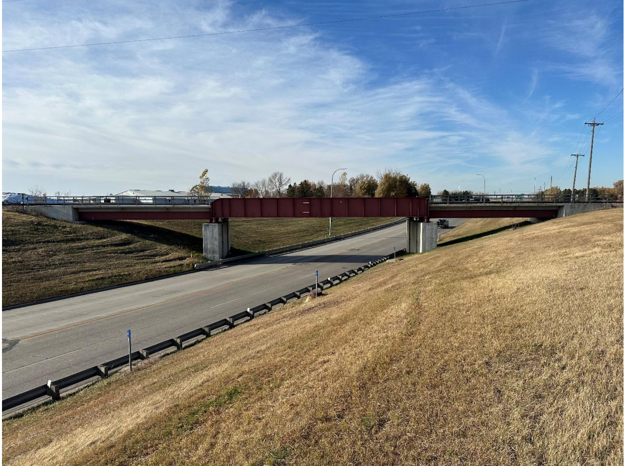
Northeast side of crossing looking West
