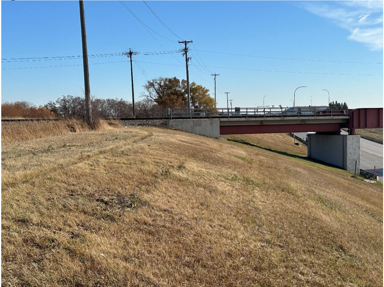
Northwest side of crossing looking East
