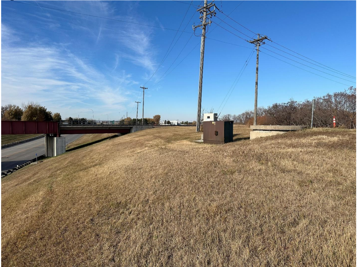
Northeast side of crossing looking West
