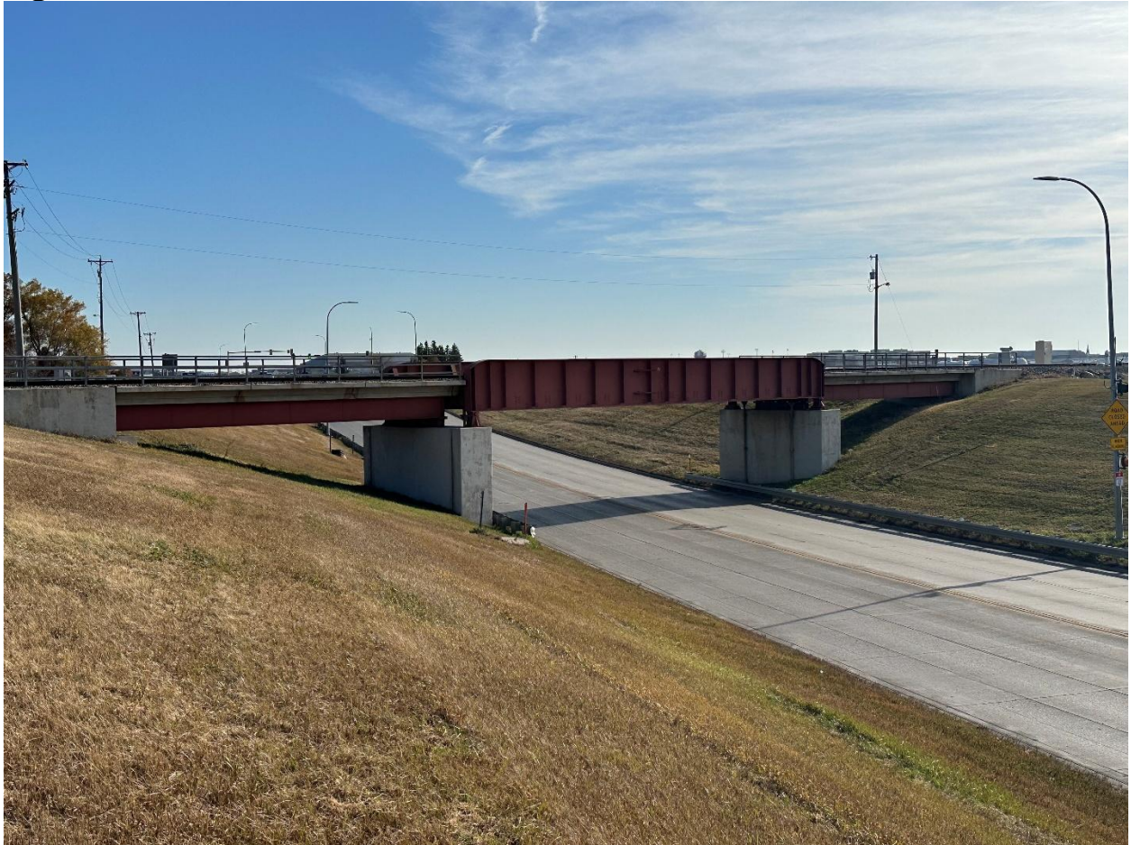
Northwest side of crossing looking East
