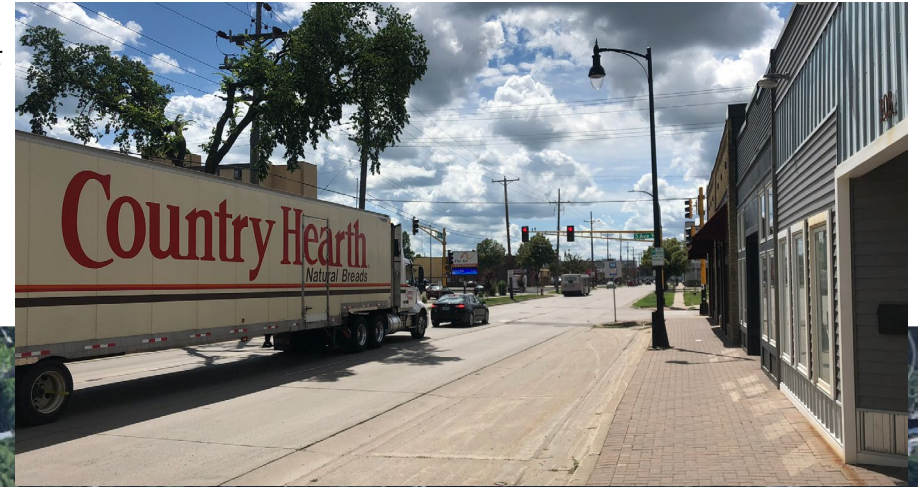
Figure 45: Retail Frontage with Pedestrian Character On-street parking and buildings fronting the street edge are present on University north of 3rd Avenue N.
