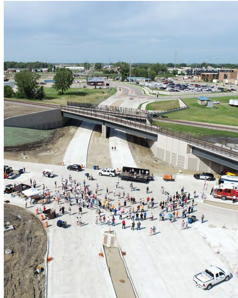
2022 Ribbon Cutting for SE Main/20 th /21 st Street Railroad Underpass in Moorhead, MN
