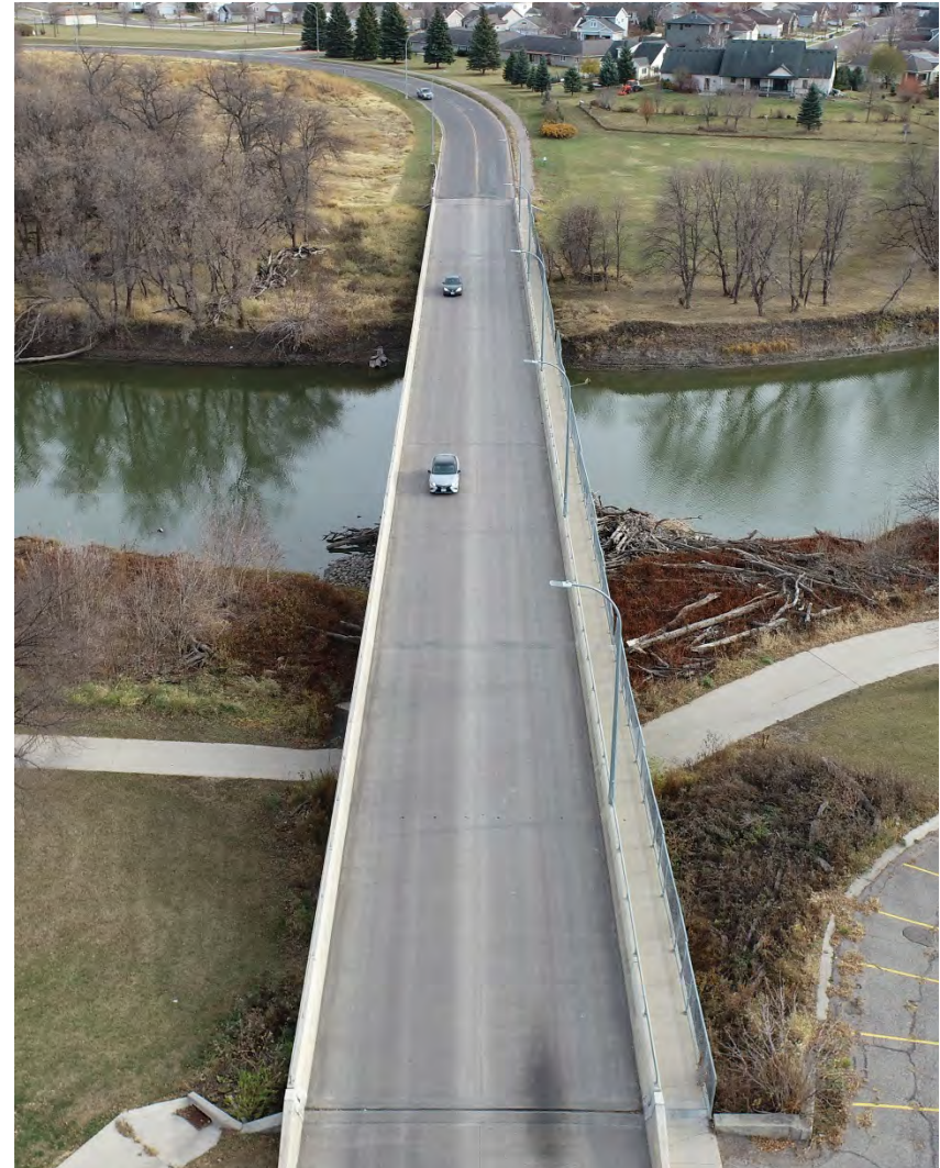
15 th Ave (Moorhead)/12 th Ave (Fargo) Bridge over the Red River
