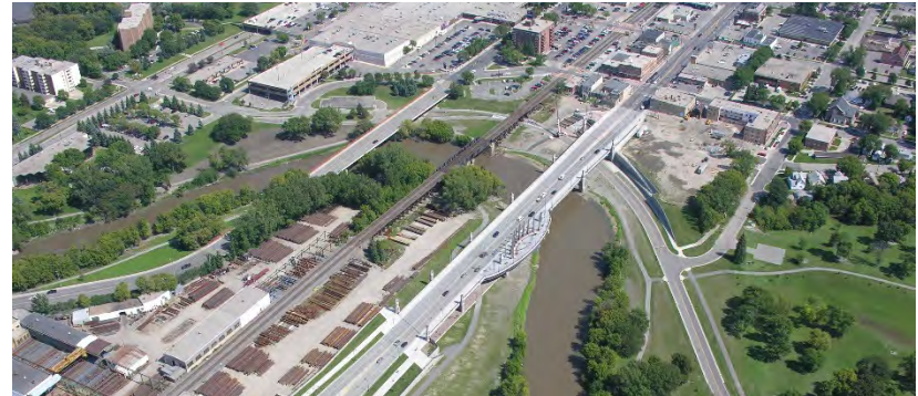
Aerial of Main Avenue, BNSF, and 1 st Avenue Bridges over the Red River
