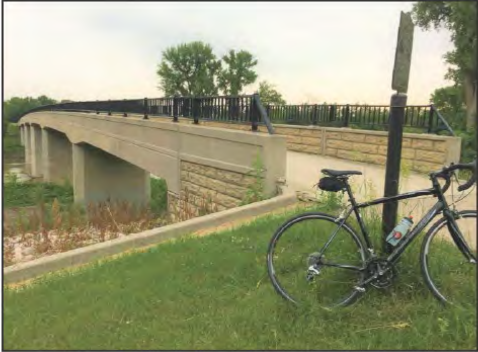
Example Image: Bicycle and pedestrian bridge in Grand Forks, ND crossing the Red River.
