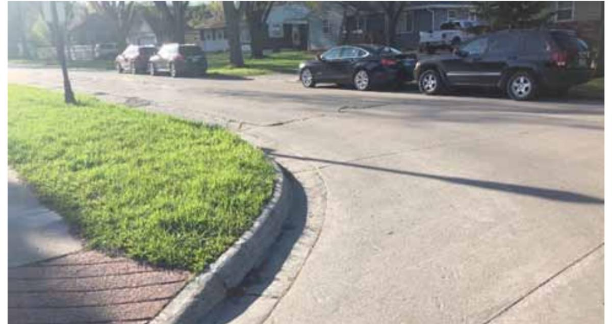
▲ The 14th Avenue S and 11th Street S intersection lacks curb cuts and pavement markings on the east side of the intersection.
