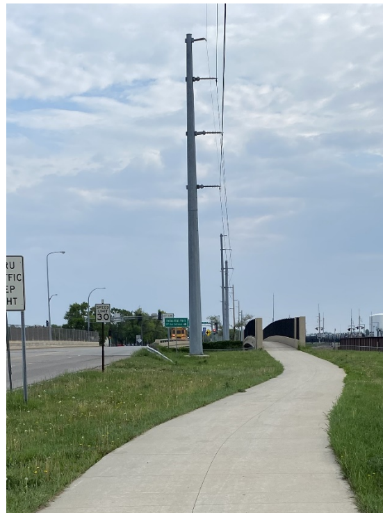
Figure 8 Power Transmission Line
