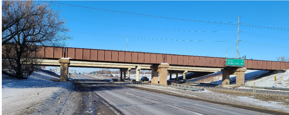
Figure 4 Existing Bridges Looking West
