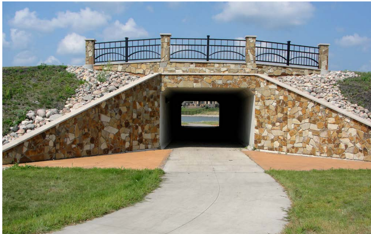
An existing trail underpass in West Fargo
