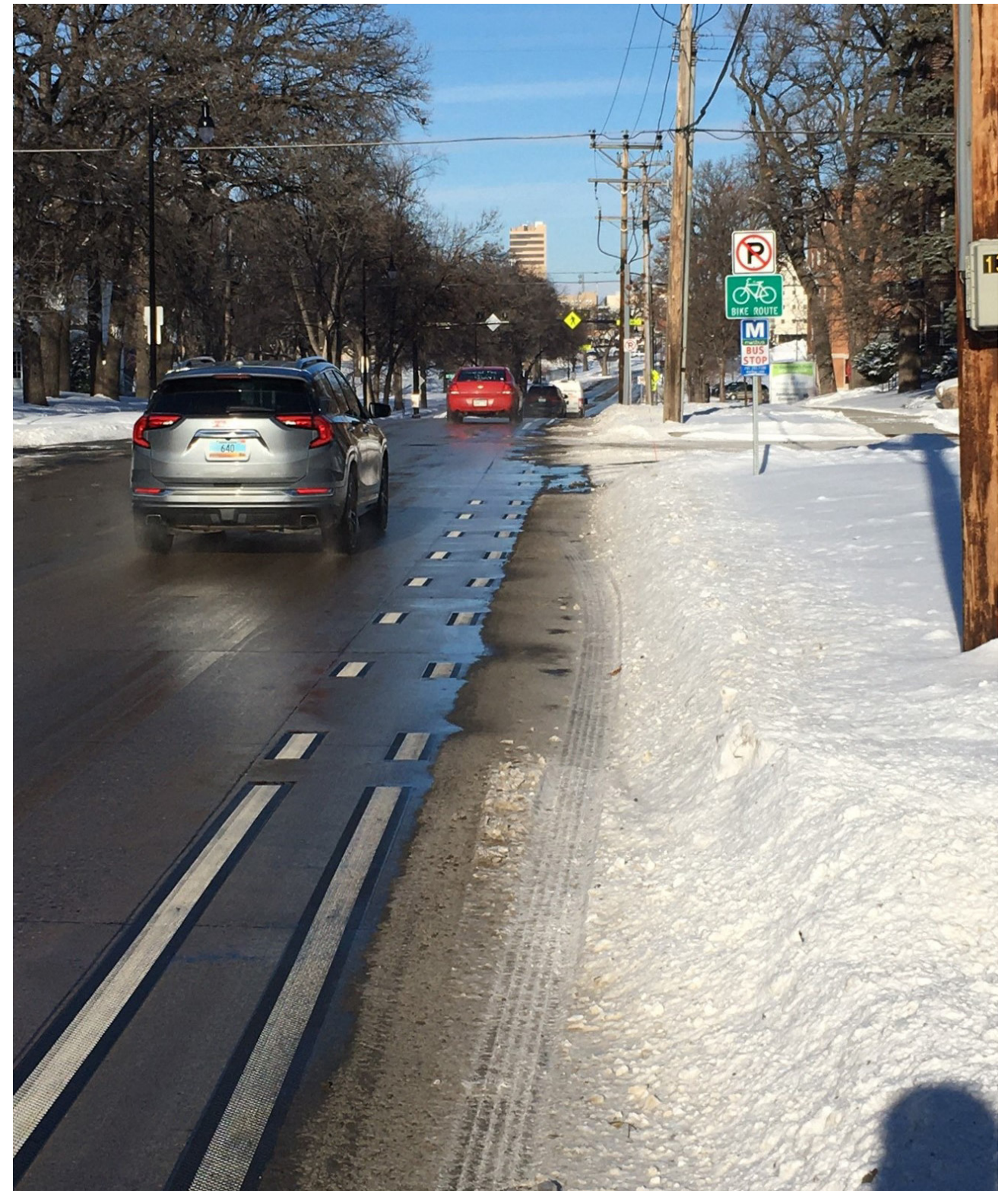
The painted bike lane along 4th St S in Fargo is inaccessible to users because snow has not been adequately plowed.
