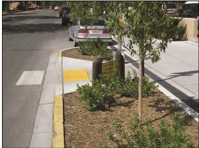
FIGURE V-8: BULB OUT AT INTERSECTION WITH GREEN SPACE AND PARALLEL PARKING
