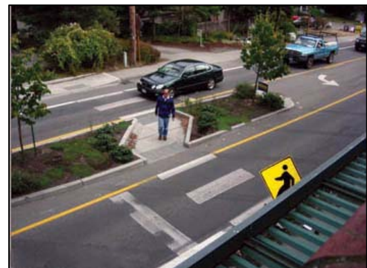
FIGURE V-7: RAISED MEDIAN WITH PEDESTRIAN REFUGE AND GREEN SPACE
