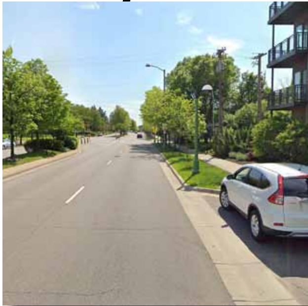
Choker narrows the roadway in St. Louis Park, MN
